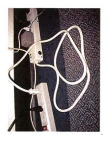
Relocatable power taps shall be directly connected to a permanently installed receptacle.
